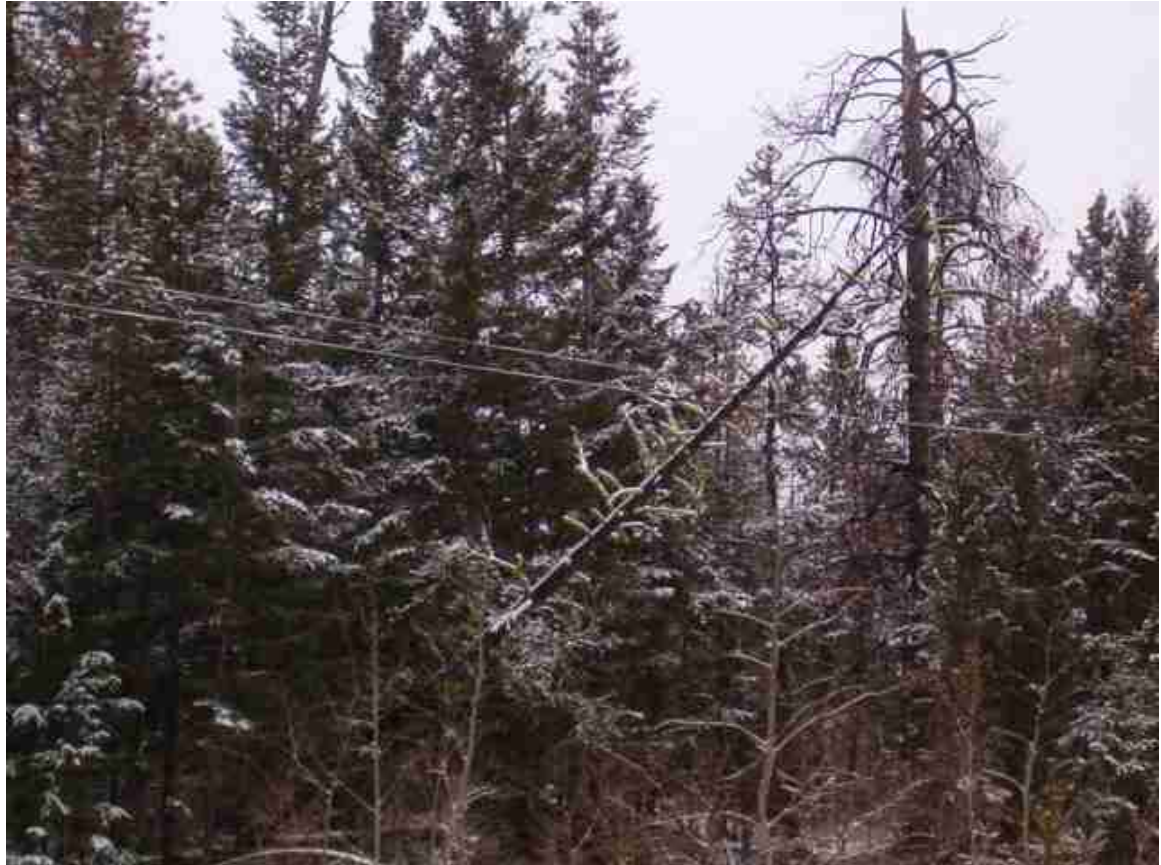
Failed pine beetle killed tree across powerlines south of 100 Mile House.
