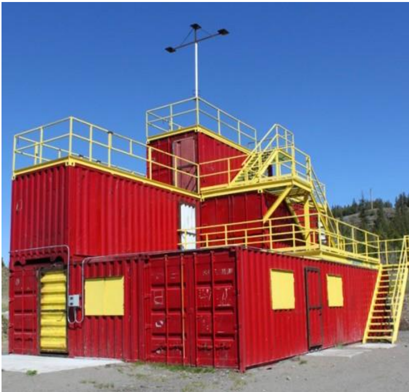
District of 100 Mile House Emergency Services Training Centre
